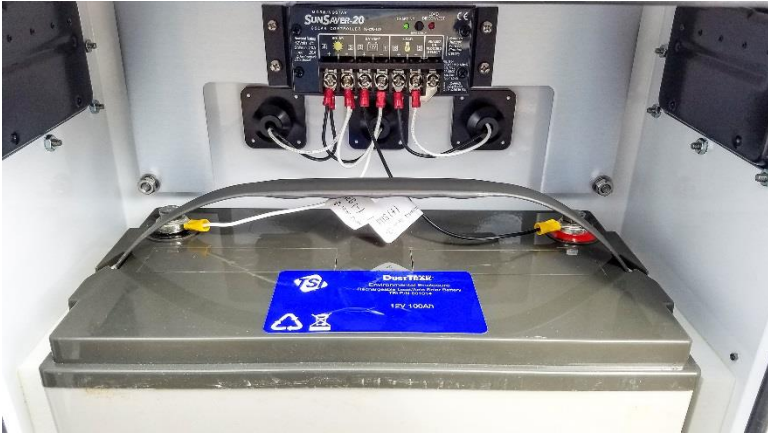
Figure 2: Install the Solar Battery and Connect to Controller
