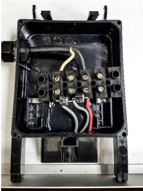
Figure 10: Attach Power Cable to Screw Terminals
