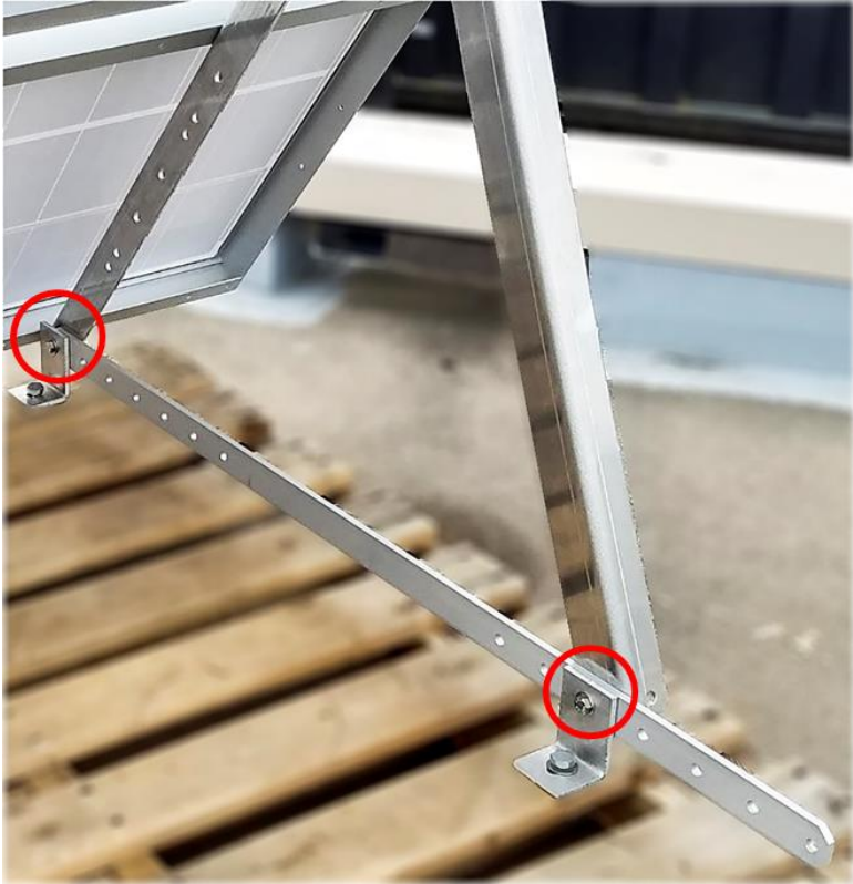
Figure 16: Fasten Two Flat Bar Pieces
