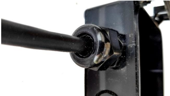
Figure 8: Tighten Nut to Create Proper Seal with the Cable
