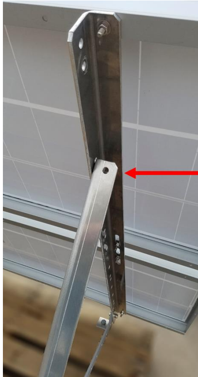
Figure 15: Attach Shorter Structural Angles
