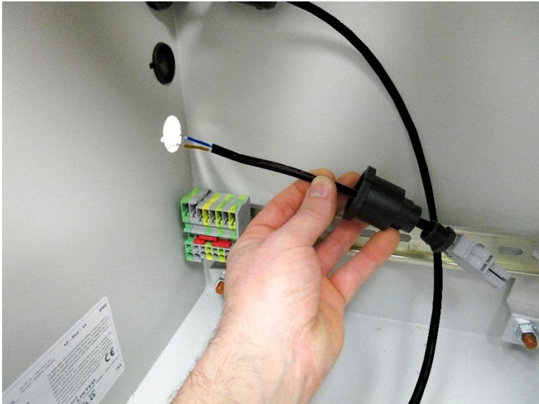
Figure 22: DC Cable Preparation
