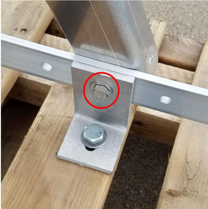
Figure 17: Fasten Mounting Feet
