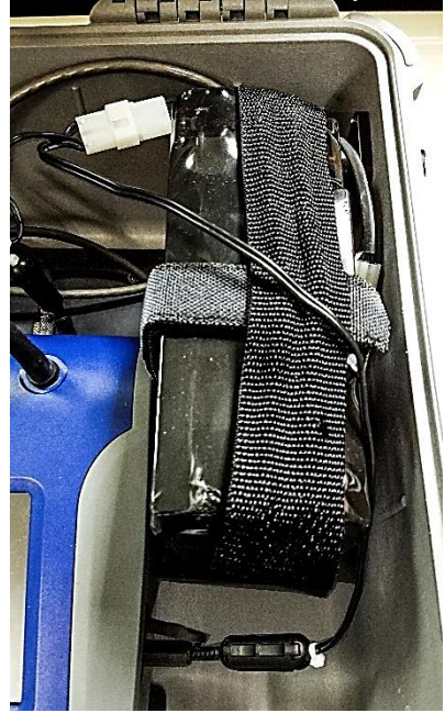
Figure 24: Internal DC Power Connections
