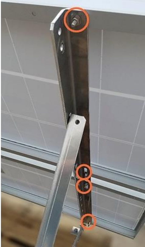
Figure 34: Assemble the Solar Cells on the Mounting Frame
