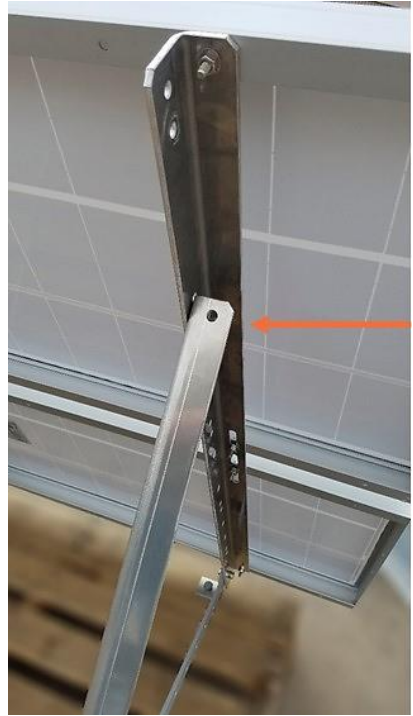
Figure 35: Attach Shorter Structural Angles
