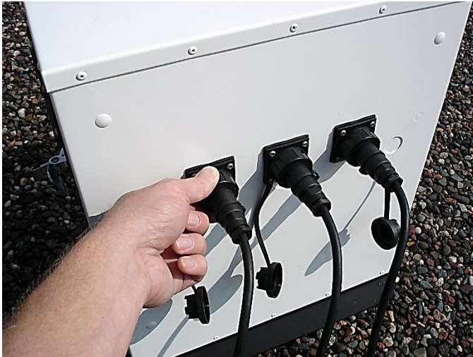
Figure 39: Connect Power from the Solar Cell Power System to the Environmental Enclosure
